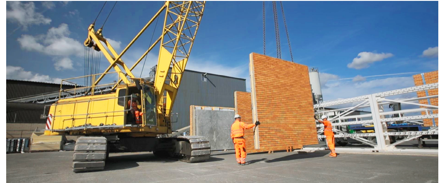
Precast panels manufactured by Forterra for HMP Five Wells
