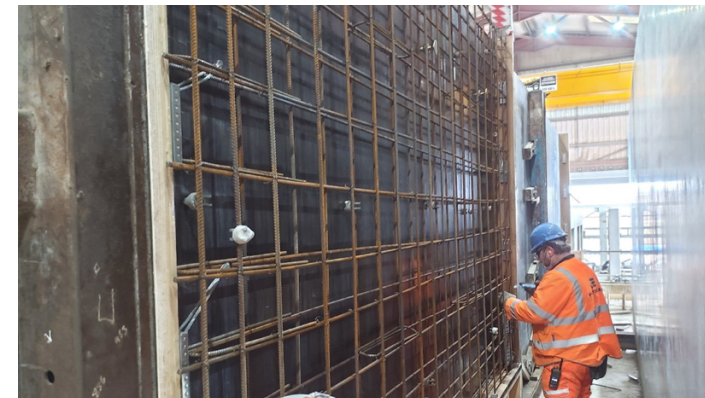
Forterra operatives preparing a precast wall slab mould
