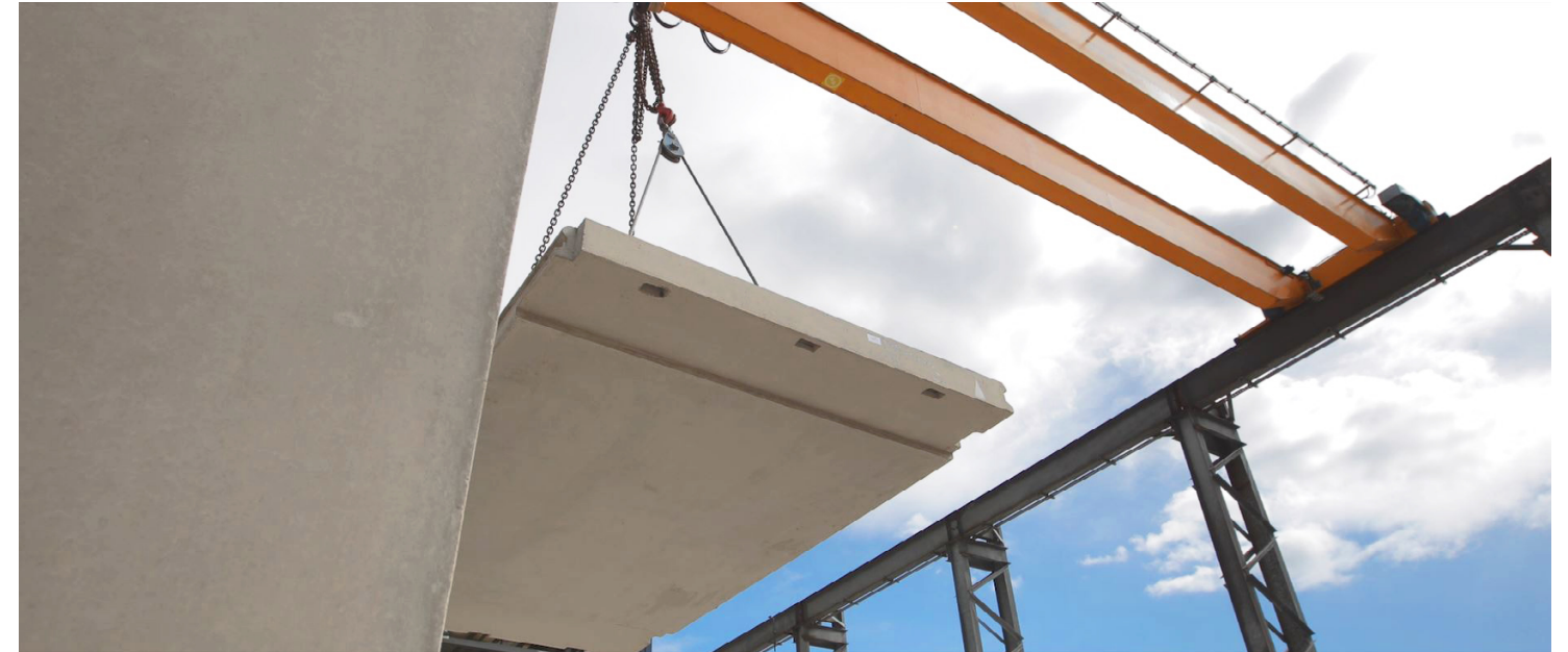
Forterra crane moving a precast panel to storage
