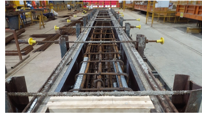
Precast column formwork
